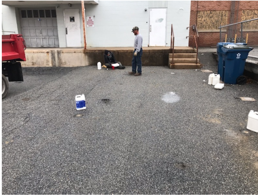
Figure 12: Soil Injection Point
